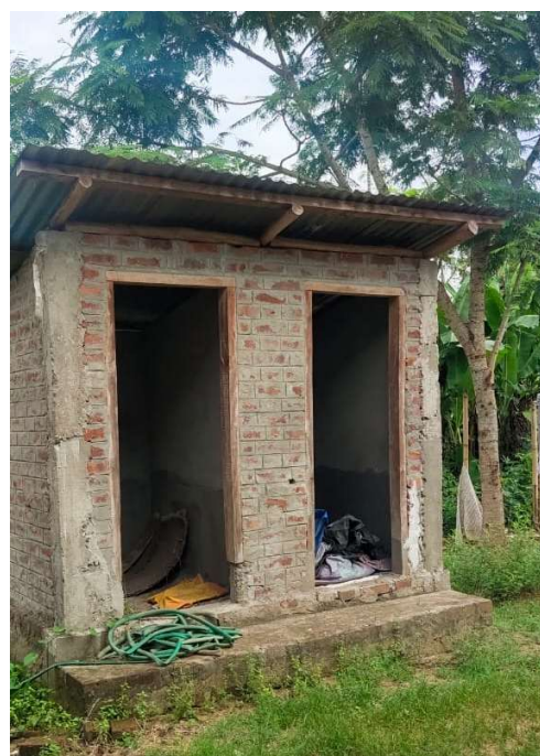
b. Under construction
