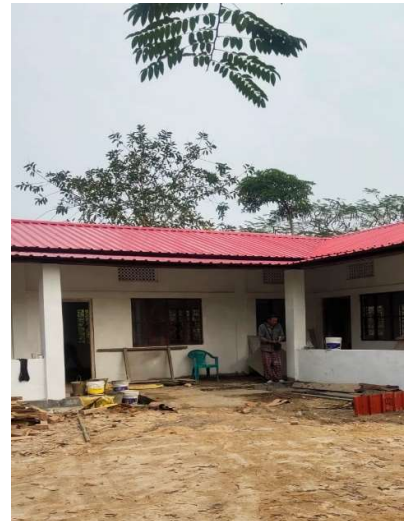
b. Extended room to be completed (Present)
