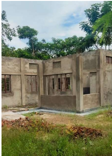
a. Extended room under construction
